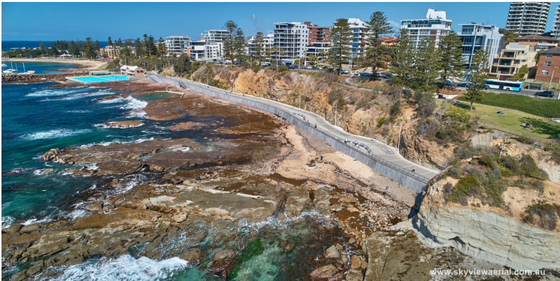
Figure 14 – Aerial Photo of New Sea Wall and Path
