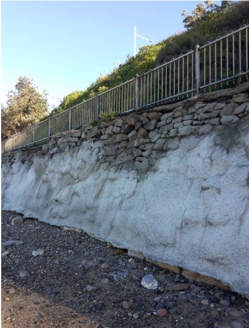
Figure 6 – Shotcrete Wall Repair
