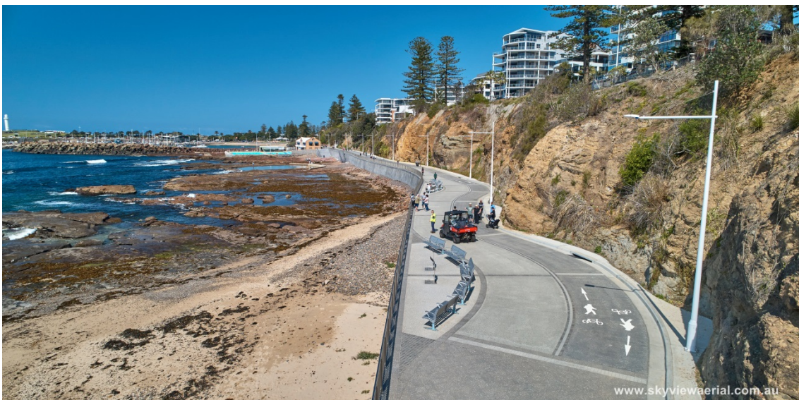
Figure 12 – Shared Path and Seating Area
