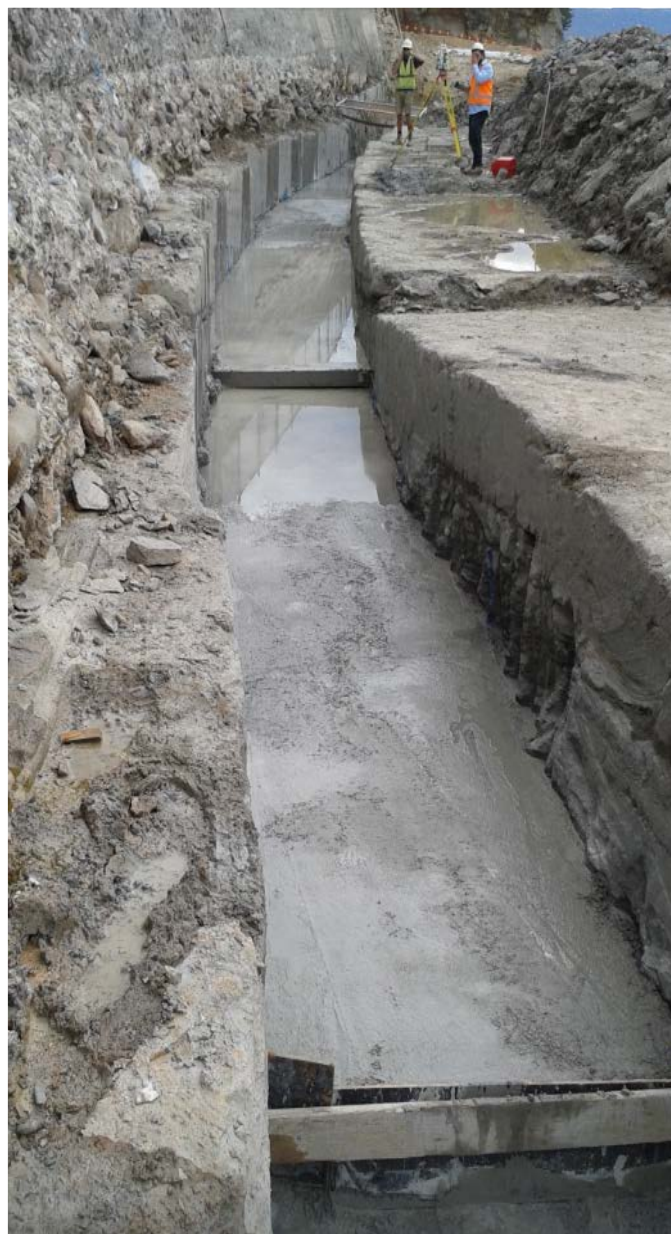
Figure 11 – Rock Trench with Bedding
