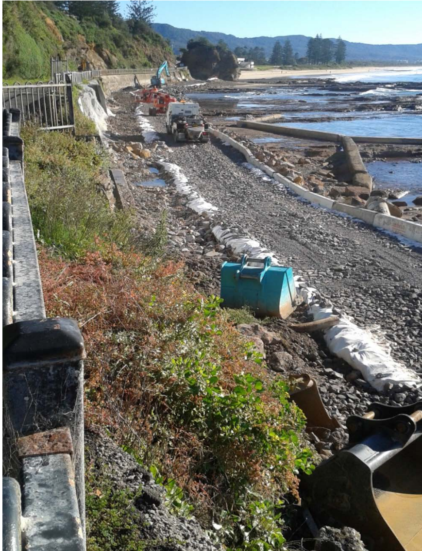
Figure 13 – Temporary Access Track
