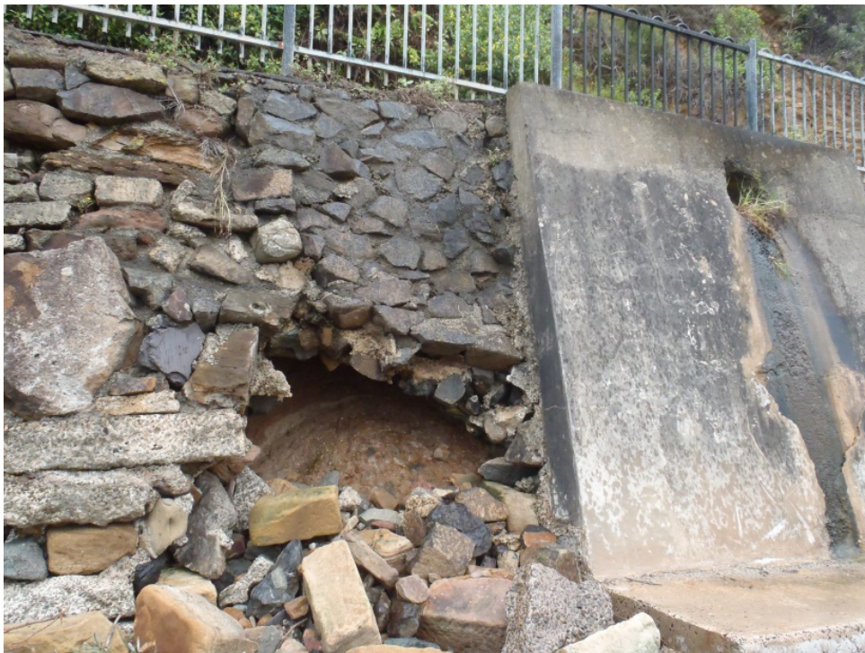
Figure 4 – Voids in Seawall 1
